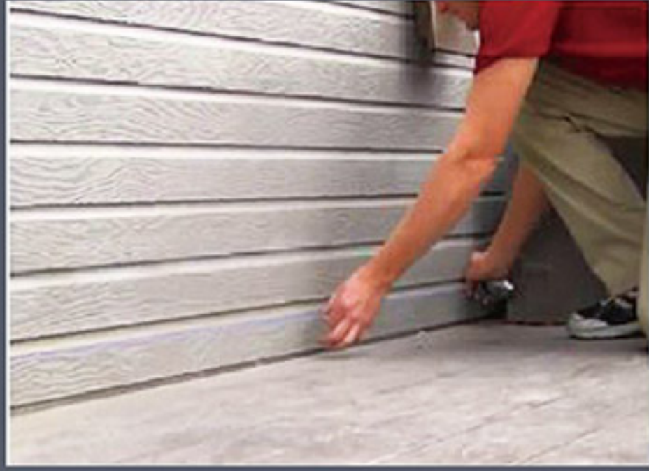
1. Level and color up the wall horizontally
