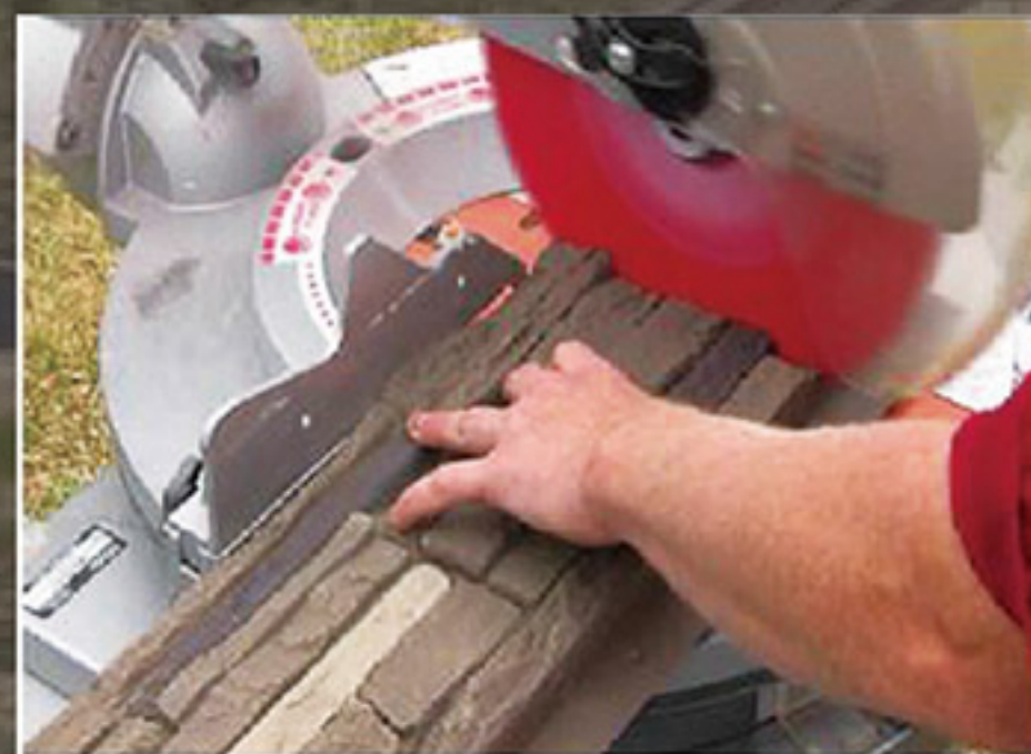
7. Cut the panel with a saw if necessary
