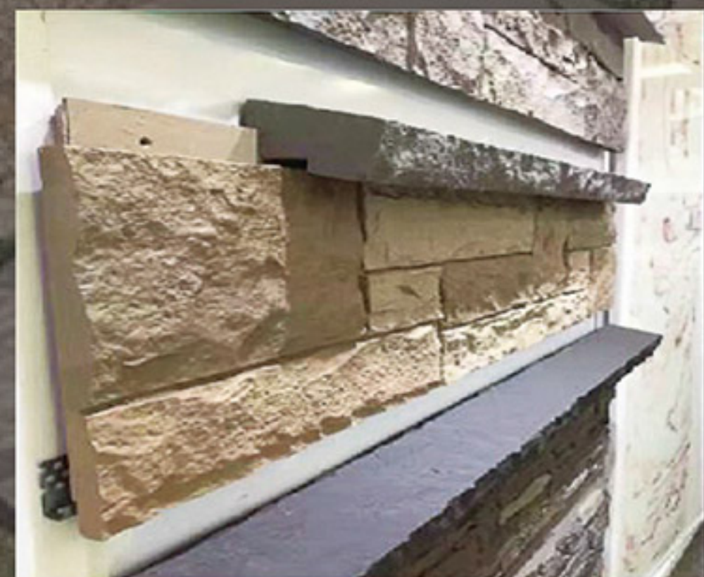
9. Upper panel interlocks with lower panel. screws are invisible.
