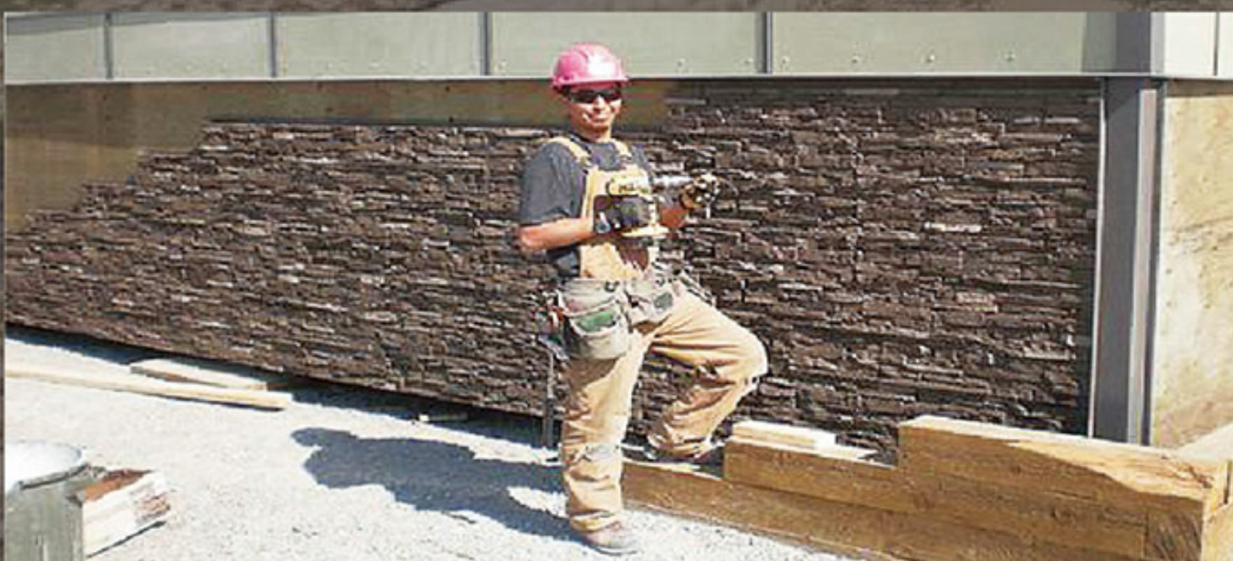
8. Drill the screw through the center of the joints to the wall.
