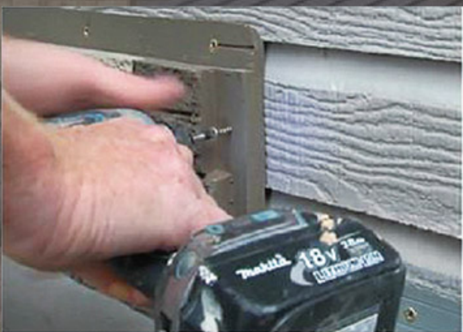
8. Drill the screw through the center of the joints to the wall.
