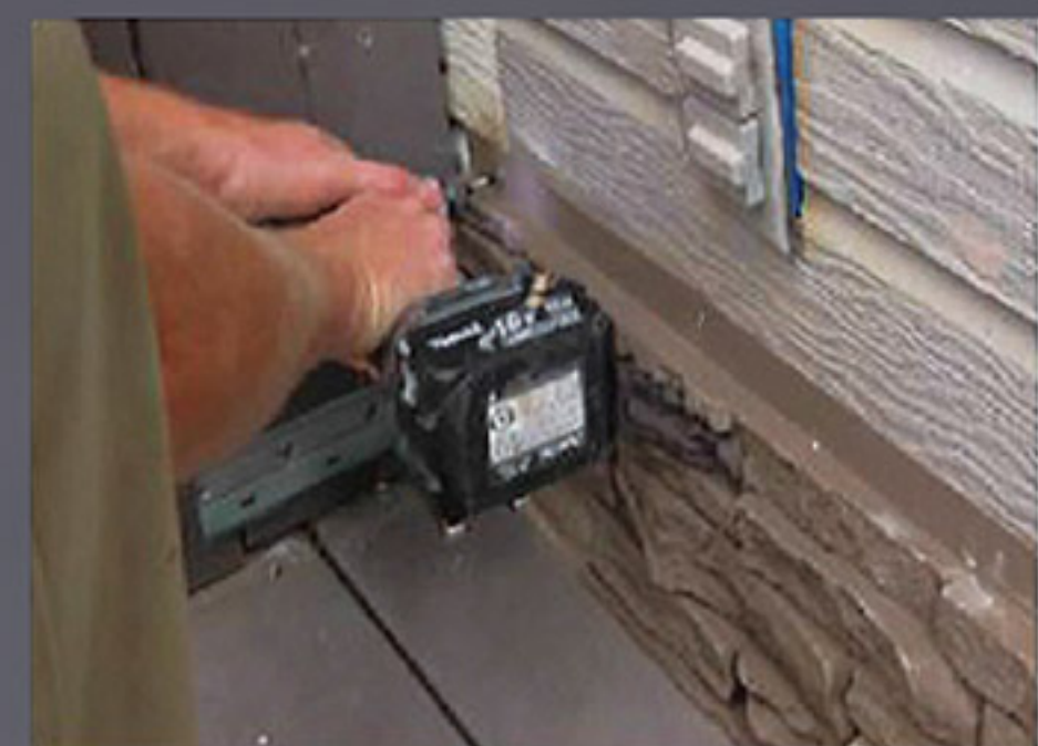
3. Install the first panel from the left bottom
