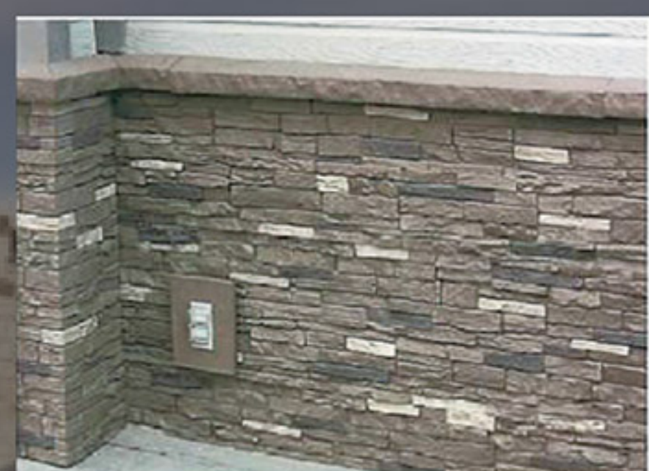
6. Keep on installing the panels, corners and top lines
