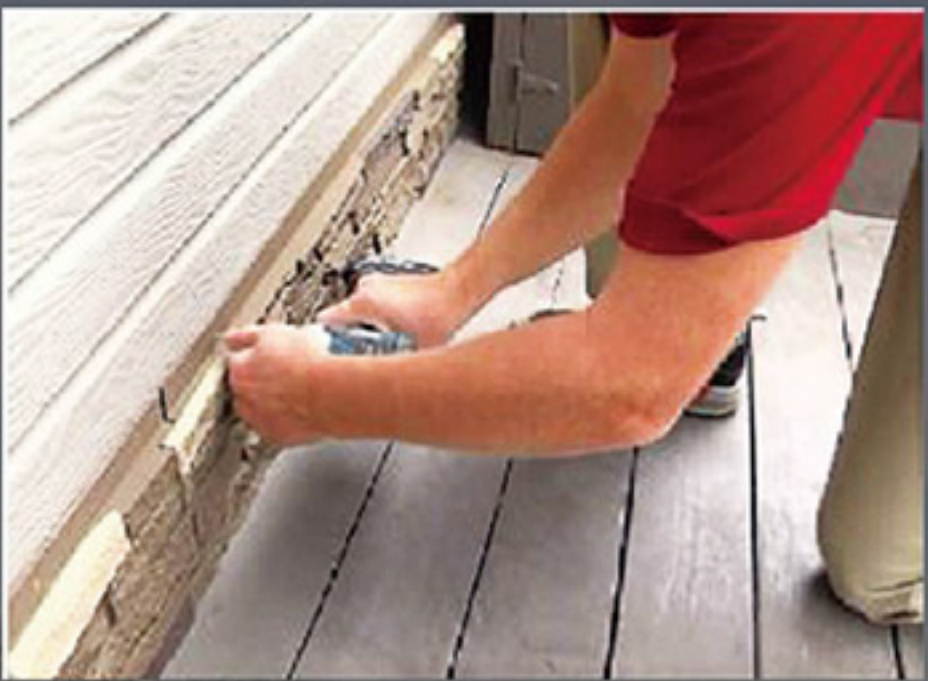
4. Lay the panels down to up, left to right, fix the panels with screws on the joints
