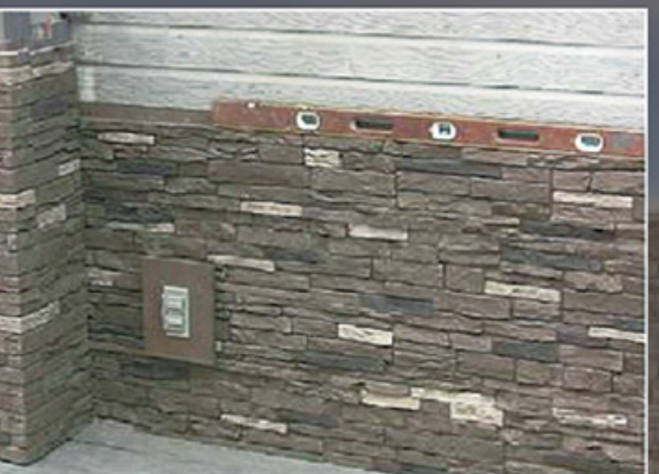
5. Check if the panels are horizontal with a level during installation
