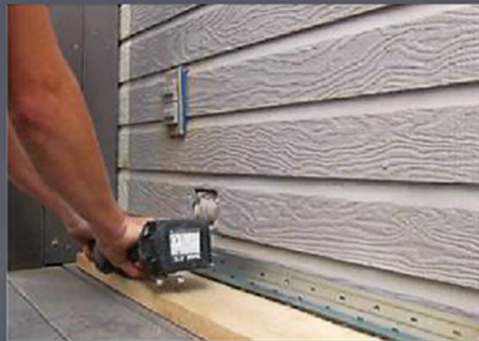
2. Put the starter strip on the bottom of the wall
